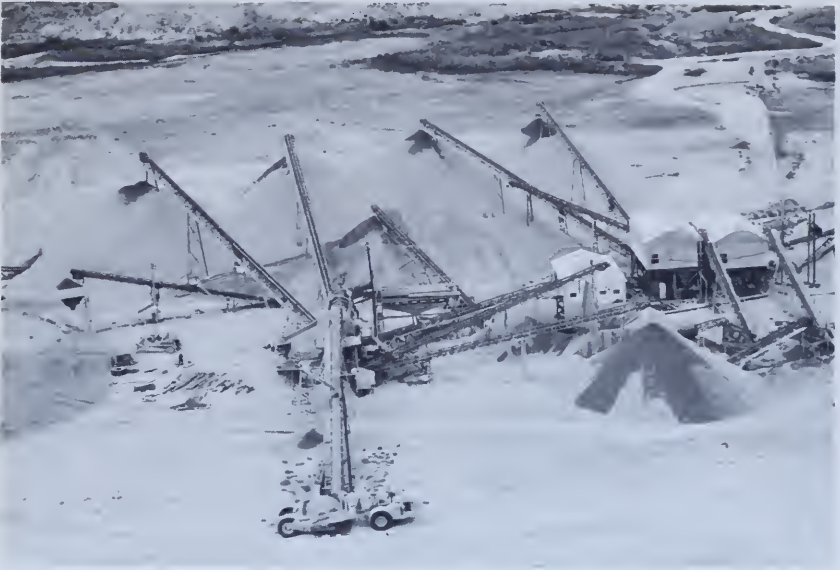
Figure 84.—Aggregate plant and stockpiles, Flaming Gorge unit, Utah. P591-421-2559.
